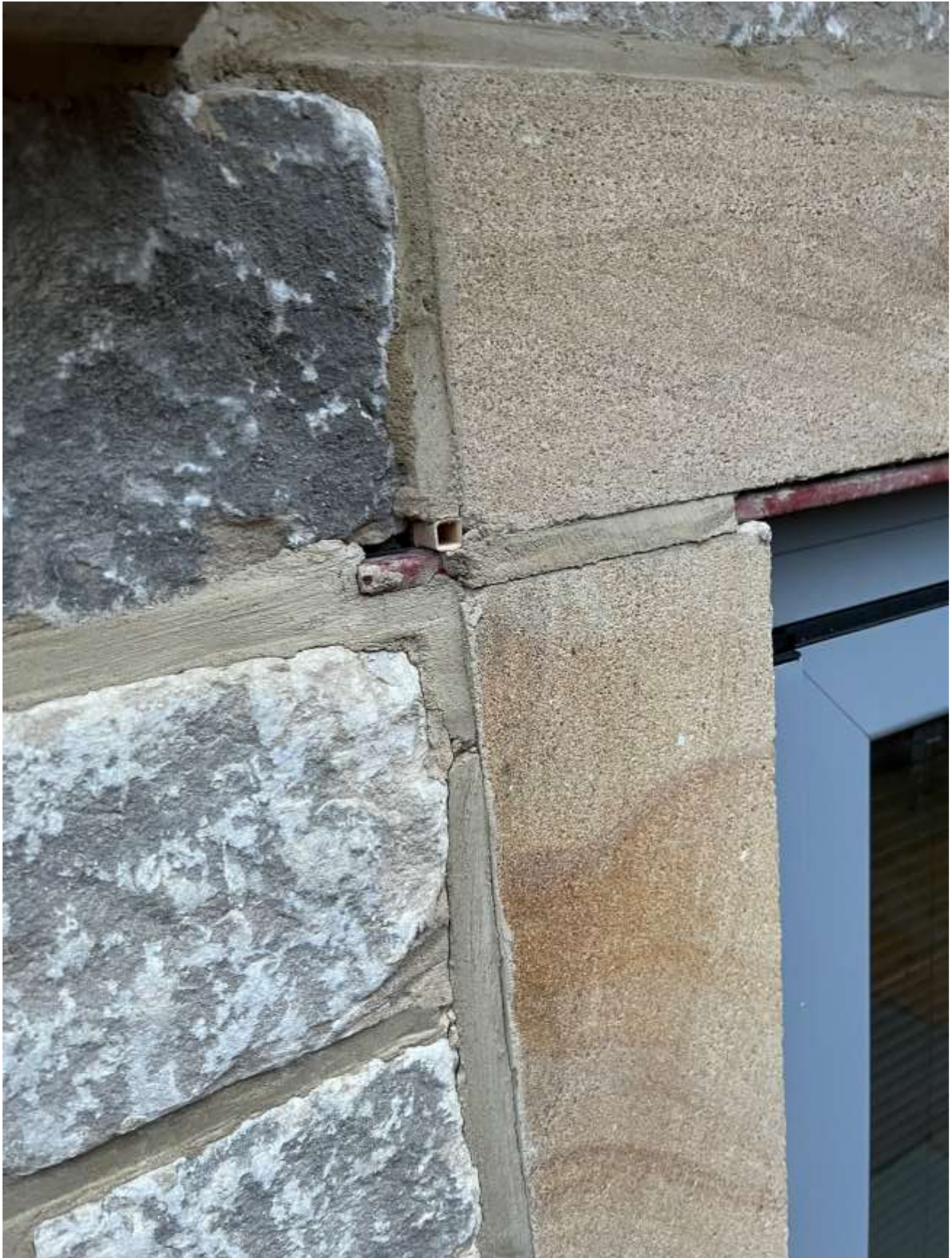
Figure 5.7 As primed steel, holes in mortar and poorly pointed. Steel left protruding preventing sufficient pointing.
