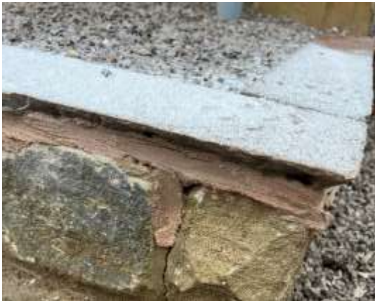
Figure 5.9 Incorrect material selection and poor workmanship
