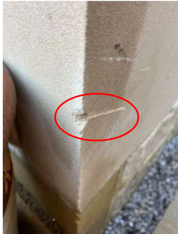
Figure 5.5 Representative images showing damage to quoins
