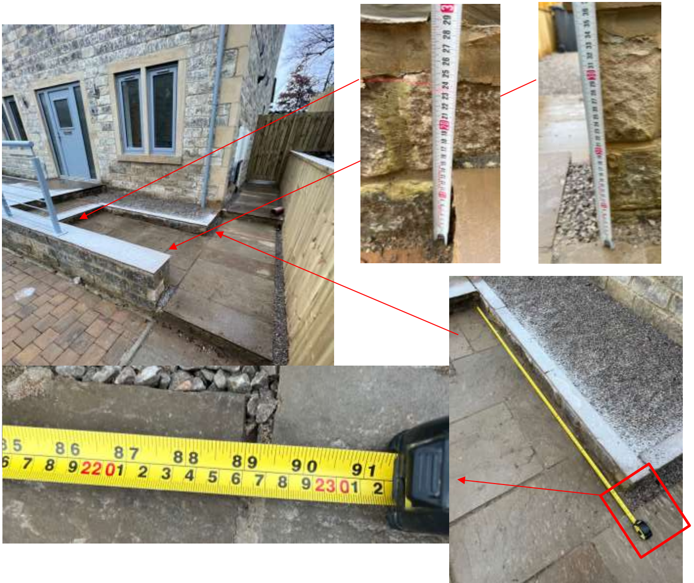
Figure 3.2: As-constructed access to Plot 25 – with measurements
