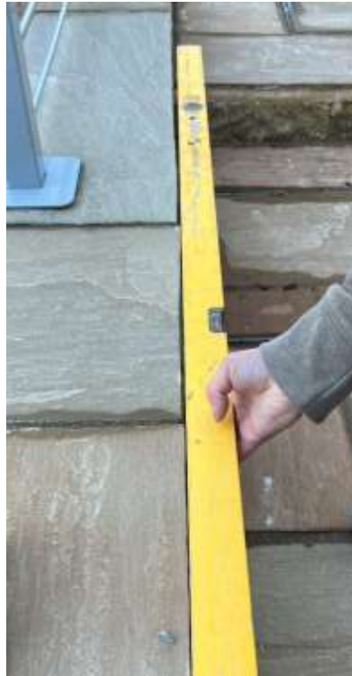
Figure 5.9 Incorrect material selection and poor workmanship
