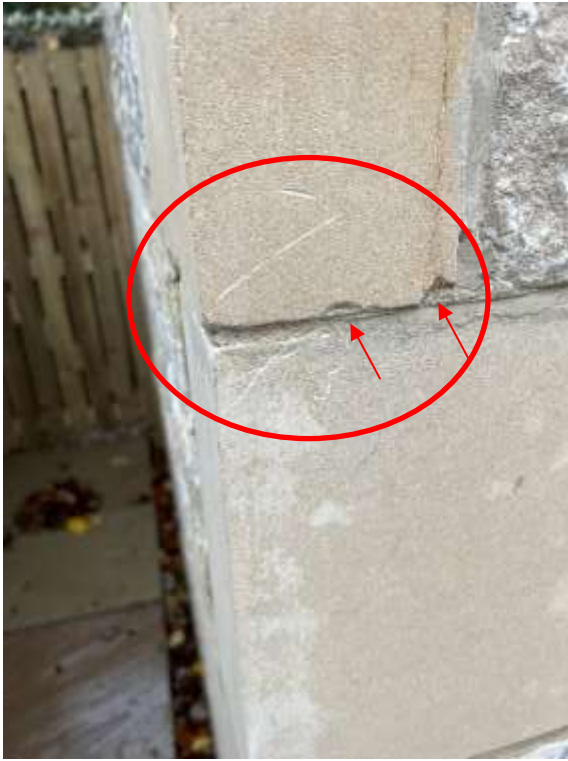
Figure 5.5 Representative images showing damage to quoins
