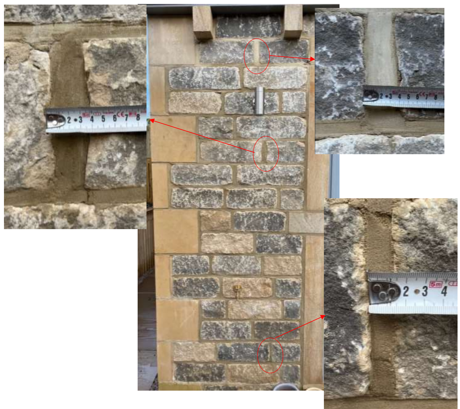
Figure 4.4 Out of tolerance perpend joints – with measurements
