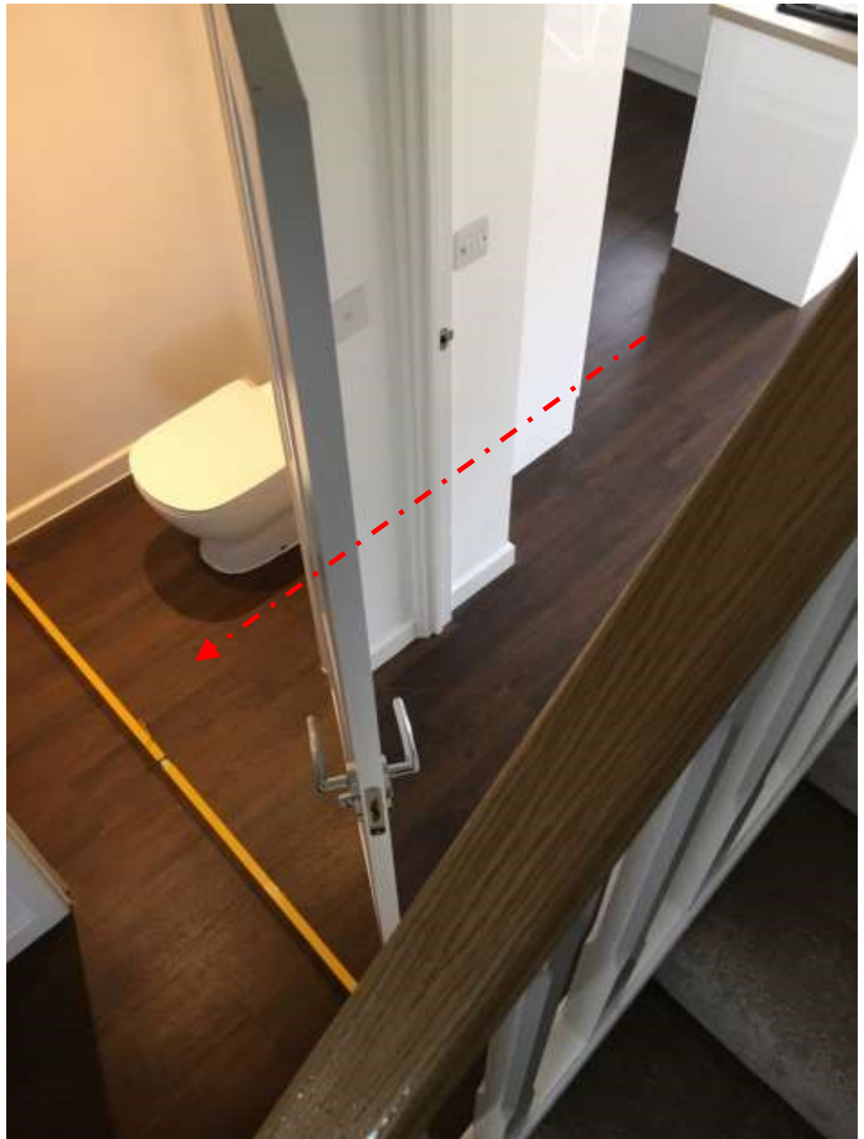
Excessive dip in floor runs through into cloakroom.
