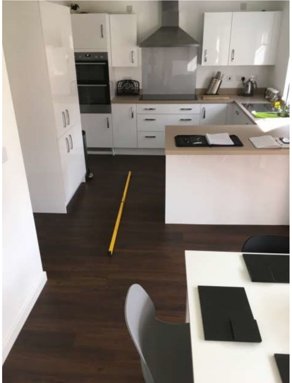
Amtico floor finish to kitchen. Excessive dip in floor to area below spirit level.
